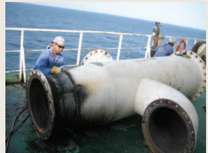
Rigging of a \phi 32" pipe from P/R to aft deck for repair
