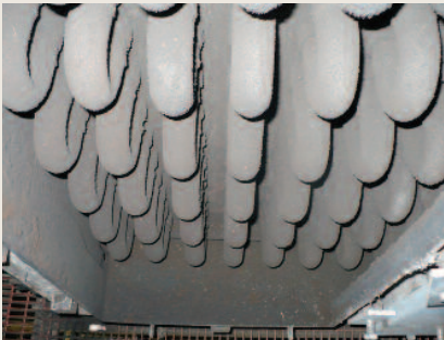
Exhaust gas economizer repair
