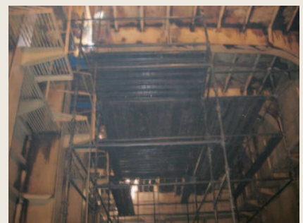
Scaffolding inside cargo tank
