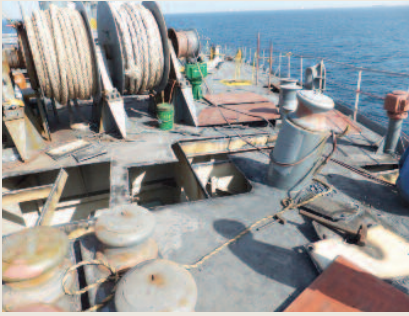
Steel renewals on the main deck
