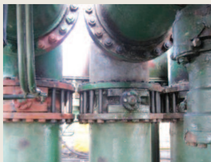
Renewal of butterfly valves on cargo line
