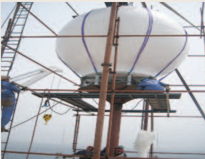
Installation of Satellite Dome
