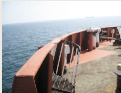
Repair of bulwark
