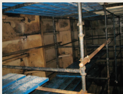
Scaffolding inside cargo tank
