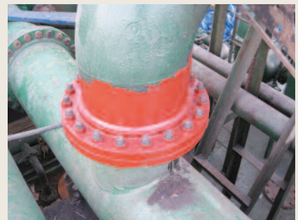
Partial renewal of cargo line on a VLCC
