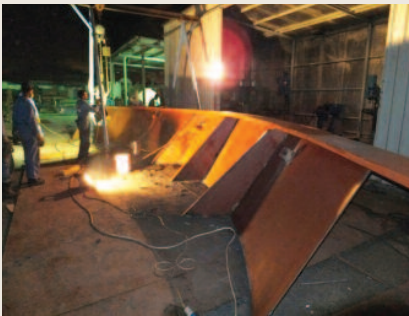
Pre-fabrication of bulwark
