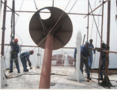
Foundation for Satellite Dome
