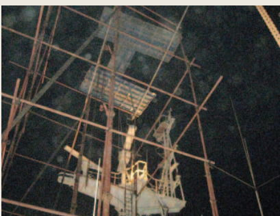
Erection of Scaffolding
