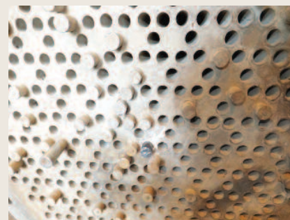
AC Condenser Repair
